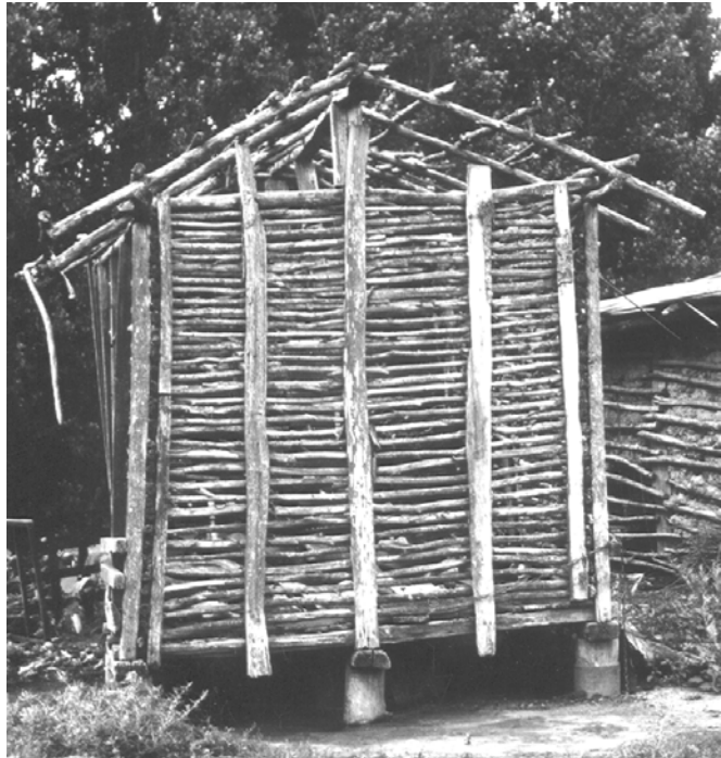
Fig. 7. A construction raised on logs from Ialomița County.
